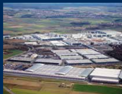
GVZ logistic centre, Germany
