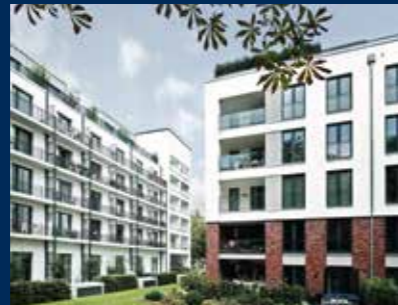
Apartment Building Hamburg, Germany
