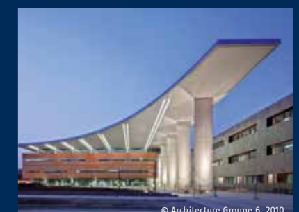
Hospital Clermont-Ferrand, France
